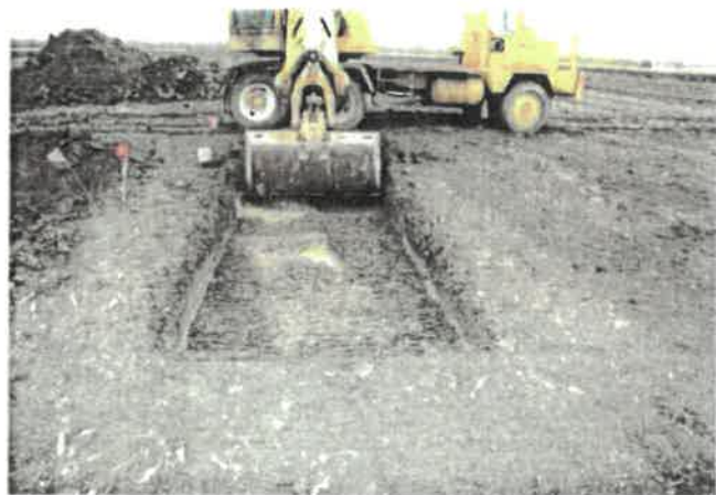
Grave Shaft Exposed During Mechanical Scraping
